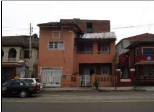
Figure 6: The insertion of contemporary architectural typologies damaged the urban image in this sector, in the formal aspect. (Mansion No. 789)
