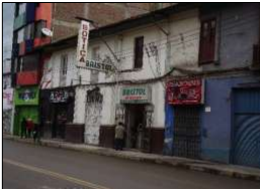
Figure 6: The change of use to which this monumental typology is subjected is evident; determined a process of deterioration and degradation in its formal expression. (Mansion No. 258)
