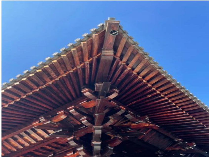
Figure 2: Detail of the mortise and tenon structure of the Gion Golden Pagoda in Shanghai
