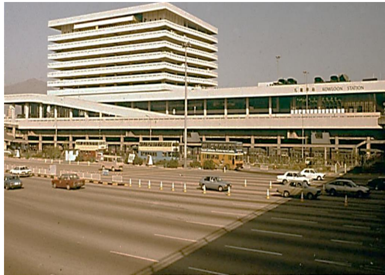
Figure 1: The Hung Hom Terminus and Multi-Storey Car Park (Li, 2023)
